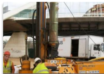
Bridge Structure Inspection
